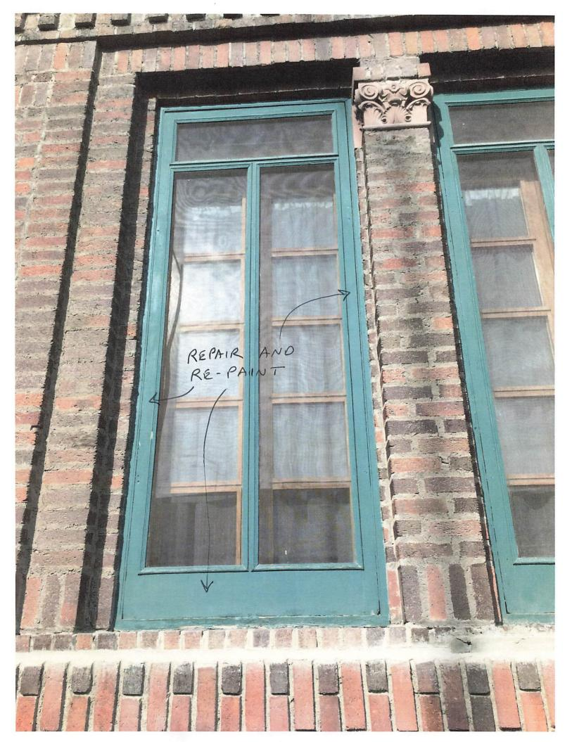
SCRAPE, FILL & CAULK GAPS REPAIR WITH WOOD ROT EPOXY AND FILCER. RE-PAINT
