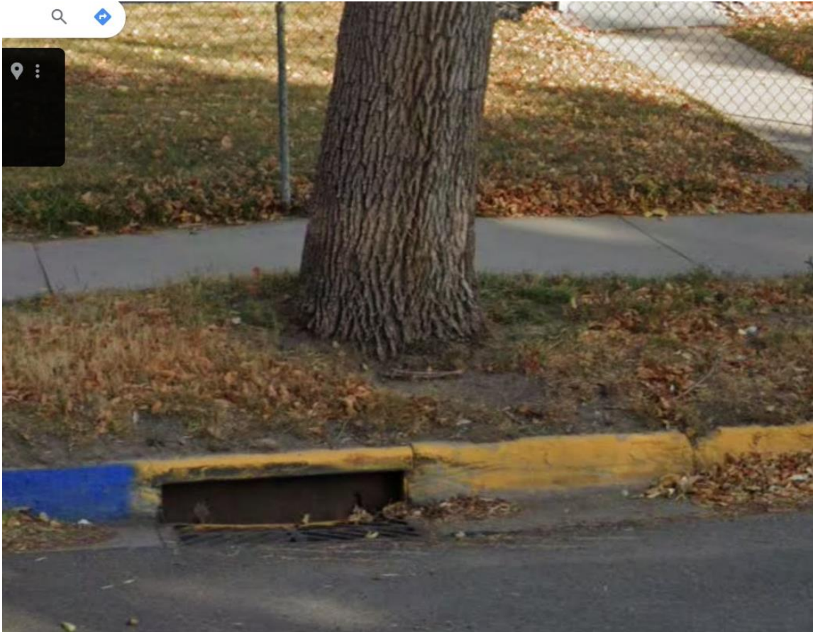
Existing stormwater inlet, north side of Stabern/Broadway intersection
