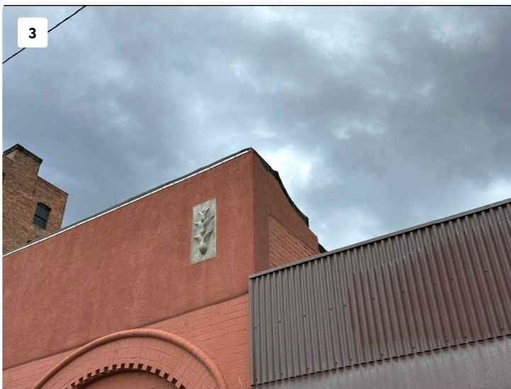
Current roof termination-addition of a parapet will provide a finished appearance
