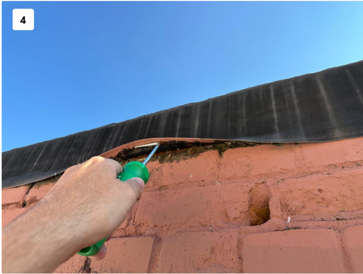
4 Current roof termination-addition of a parapet will provide a finished appearance
