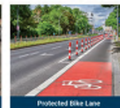
Protected Bike Lane
