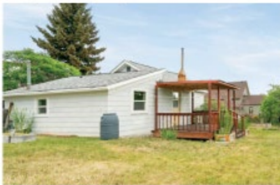
Photo of the back of the addition and the deck with roof.
