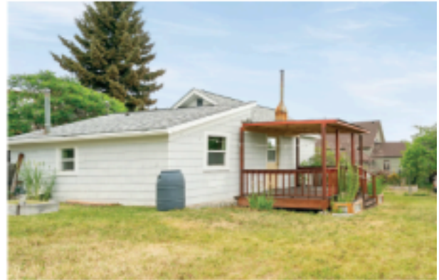
Photo of the back of the addition and the deck with roof.
