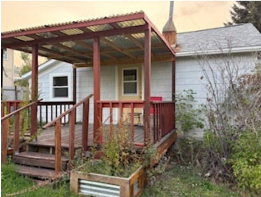
East side of house facing Davis St.
